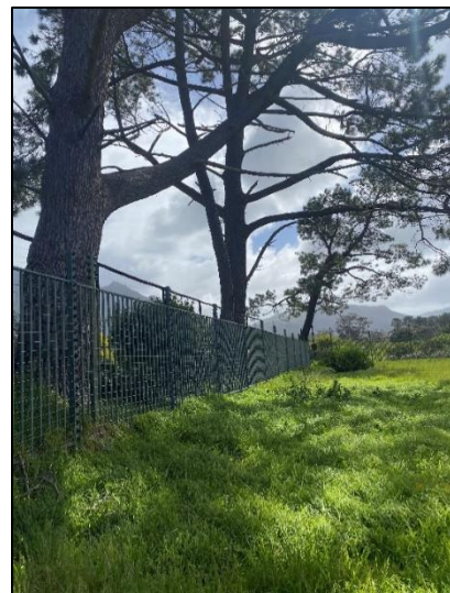
Figure 7. Large tree overhanging the electric fence at Steenberg Green.
