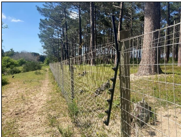
Figure 6. Broken electric fencing at Tokai Picnic site.
